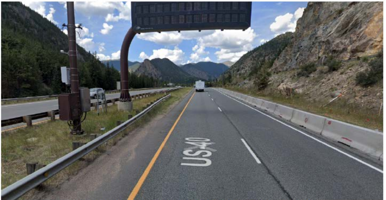
Figure 5: WAL-E location 3 (39°45'44.32"N, 105°38'39.76"W)
